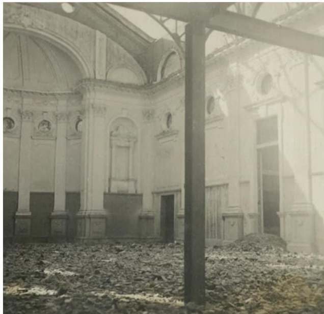
HKU Interior of Great Hall - half right view. Photo: Public Records Office, Government Records Service.
