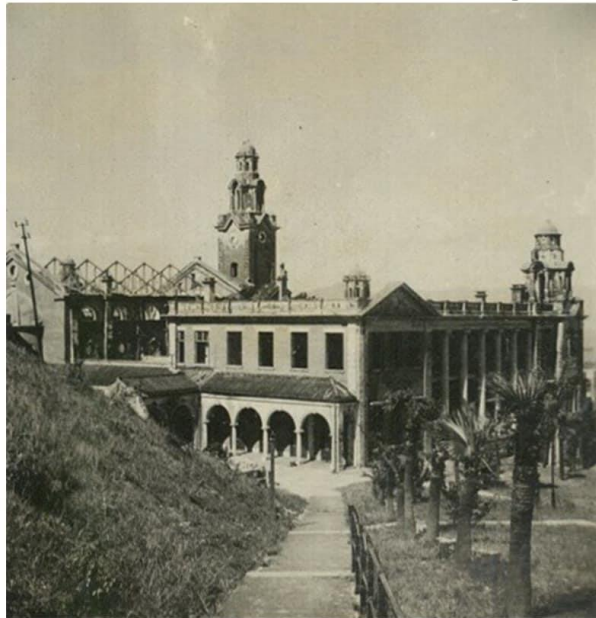
HKU Main University Building - showing damage to roof of Great Hall. Photo: Public Records Office, Government Records Service.
