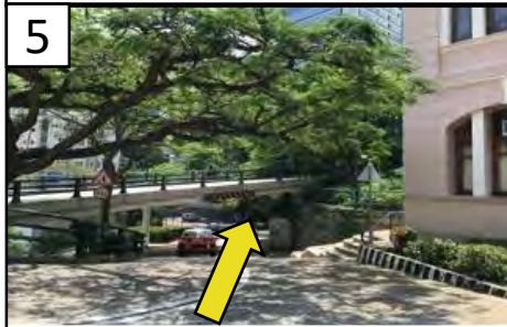
5 Walk down the slope.
